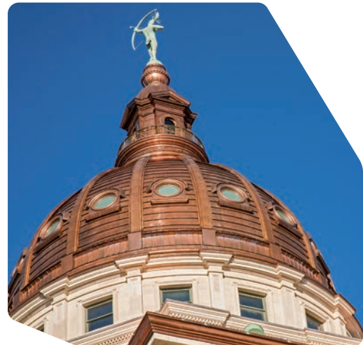
Restoration of Kansas Statehouse (USA)
